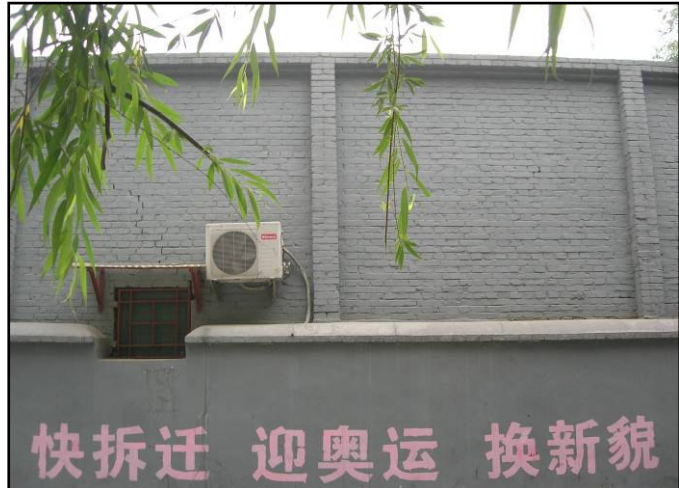
Dongchang hutong: text reads "Demolish quickly, Welcome the Olympics, Switch to a New Look."
