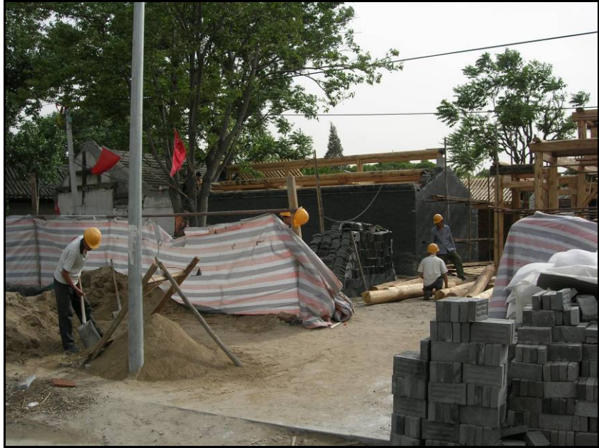
Demolition and reconstruction in Xianyukou
